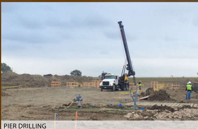
PIER DRILLING
